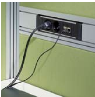
Wiring: Power and data flow always in the right place.
